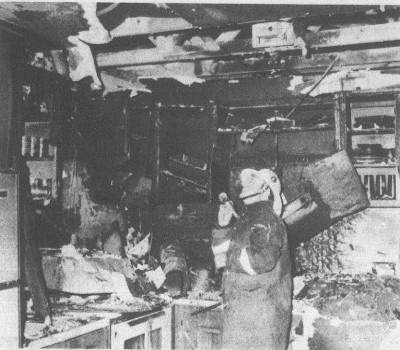
INSPECTS DAMAGE ... Chief Melvin Fussell inspects the damage in the kitchen area of the home in which the Ed-
