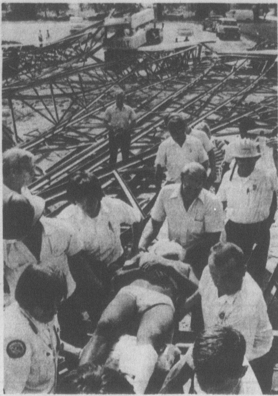
CARRIED FROM WRECKAGE — Construction worker William Rivers is carried from the scene to a waiting ambulance after the steel framework for the Forest Heights Baptist Church in Tallahassee, Fla., collapsed. Rivers was pinned beneath the wreckage. A total of eight persons were injured in the Wednesday mishap and the cause of the collapse was not immediately known. (AP Wirephoto) — Copyright Photo by Dan Stainer of the Tallahassee Democrat, 1977.
