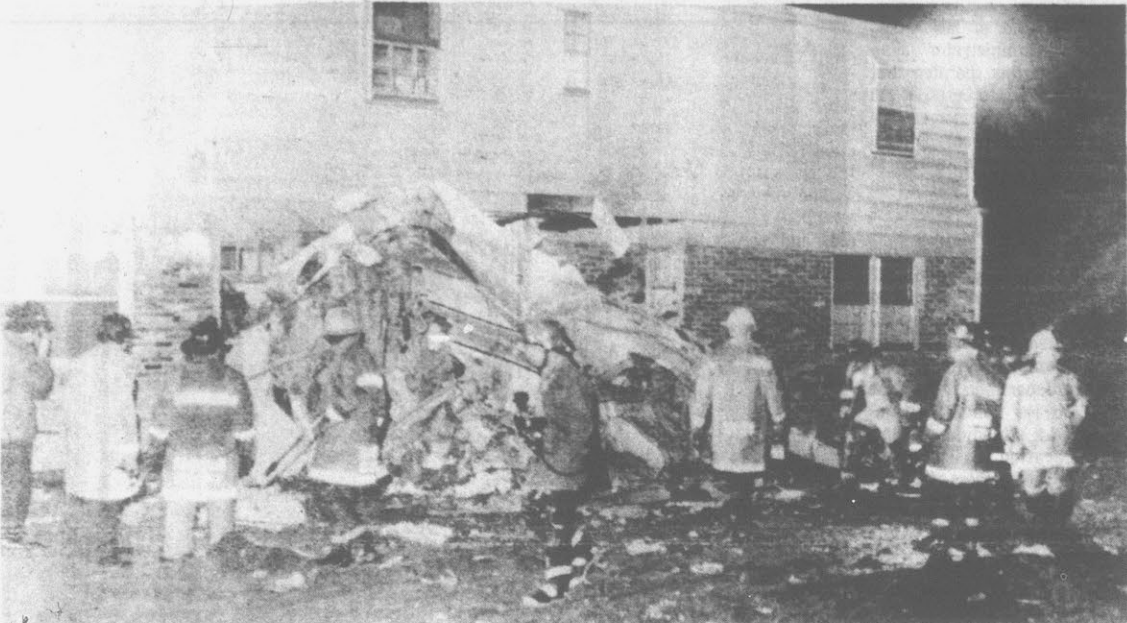
CLOSE CALL — A section of a twin-engine jet lies against a McLean, Va., home after the craft crashed killing three persons aboard Thursday night. A wing and gas tank hit a nearby home and
