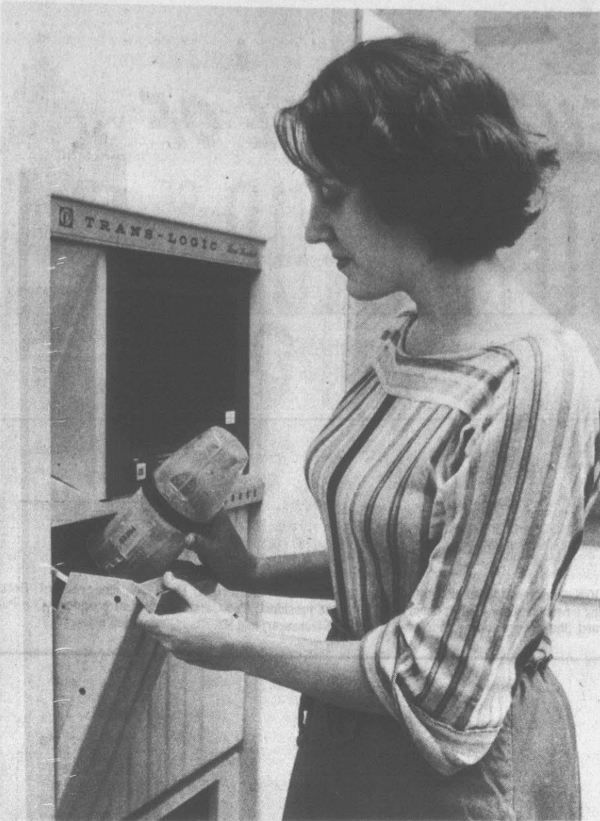
PNEUMATIC SYSTEM... Pam Burke, secretary in the office of hospital construction manager Ralph Hall, demonstrates the use of the pneumatic transporting system that will be available at the new medical complex. (Reflector Photo By Tommy Forrest)
