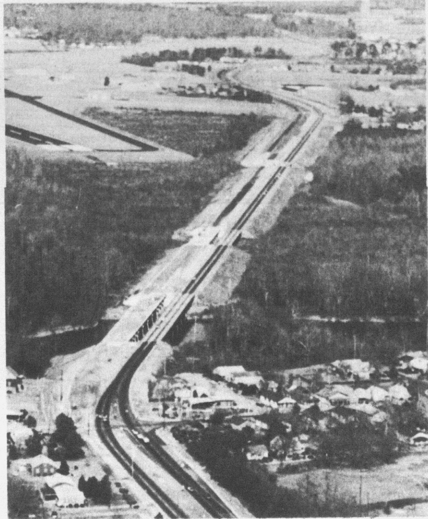
Completion By October
