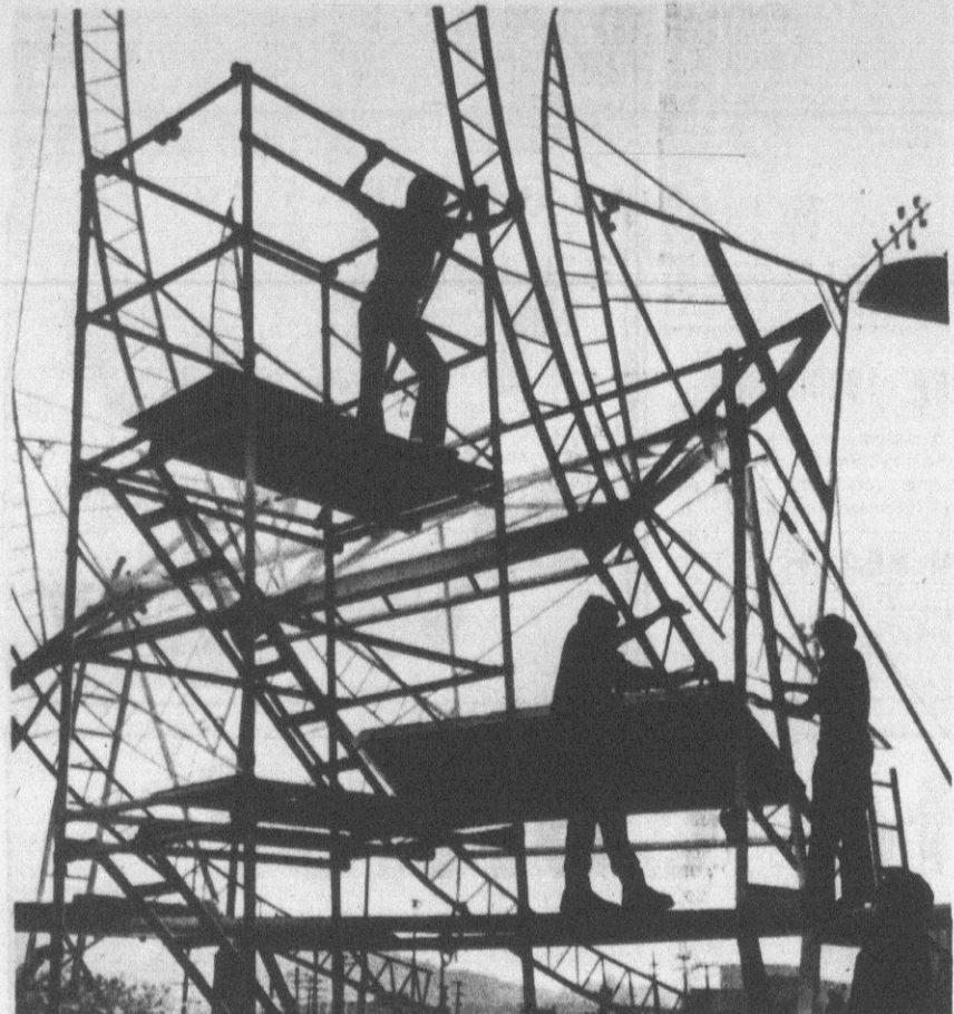
BUILD SOLAR GENERATOR — This 34-foot solar dish and electrical generator being constructed by JPL engineer Howard Broyles and high school students, will be used on Pitcairn
