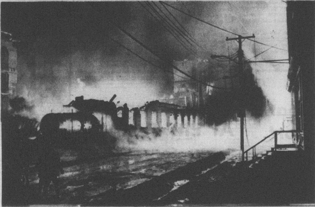
Manufacturing Complex Burned
