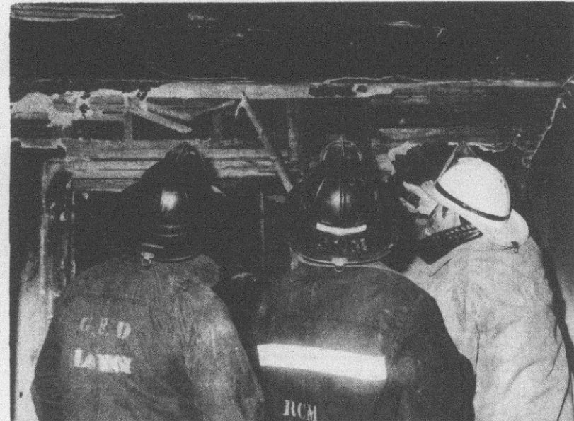
SATURDAY FIRE — Greenville firemen look over damage caused in a 9:15 p.m. fire Saturday at 404 South Jarvis St. Officers reported the blaze heavily damaged the heating plant room and caused heavy smoke damage to the rest of the wood-frame dwelling. Fire officials said cause of the blaze has not been determined.
