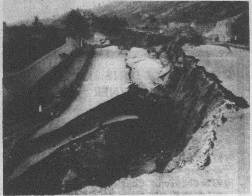
ROAD IN RUINS — The road which winds at the foot of Giuliano Mountain in Sicily appears almost entirely destroyed by one of the landslides which hit several areas of Sicily in the past days. The landslides, caused by continuous
