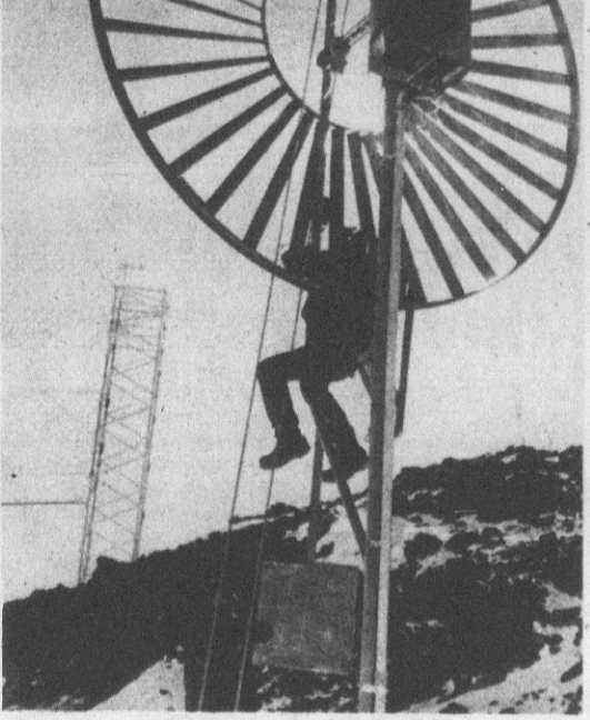
Using The Air Waves — Workman inspects 12-foot wind turbine atop 13,000-foot peak overlooking Copper Mountain, Colo. The turbine supplies power for transmitter that gathers live television signals and rebroadcasts them to the community. The wind turbine powers the transmitter at a savings of some $75,000 over commercial power sources and is the first such installation in the United States according to Ray Bishop, designer of the system (AP Wirephoto)
