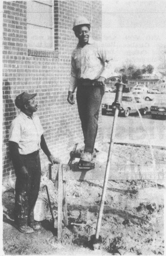
AN UNLIKELY PLACE... for a hand pump, it would seem, is the 200 block of East Third Street, but Greenville Public Works employee Frank Jones spent much of Friday afternoon welding its handle. He said there was an underground water tank that had to be emptied and removed before the sidewalk could be laid. His co-worker Braxie Cox (left) assisted. (Reflector Photo by Carol Tyler)
