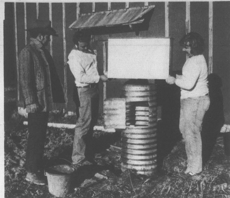
INSTALL OBSERVATION WELL — James Galloway, left watches Gene Baker, center, and Joe Riggsbee, right, hydrologic technicians, install
