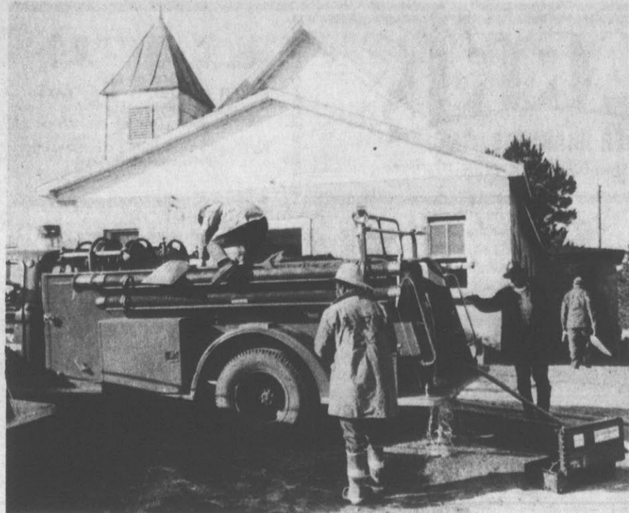
FIRE . . . damaged St. Paul Disciples Church of Christ on East Avenue in Ayden Sunday morning. The blaze was contained in a room at the right rear of the sanctuary, Ayden firemen said. They believe it was started by a gas heater in that room. (Reflector Photo By Tommy Forrest)
