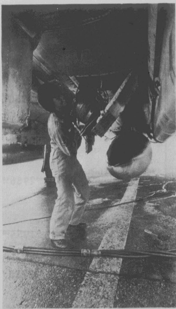
Heave ho, oxygen converter is stowed into F-4.
