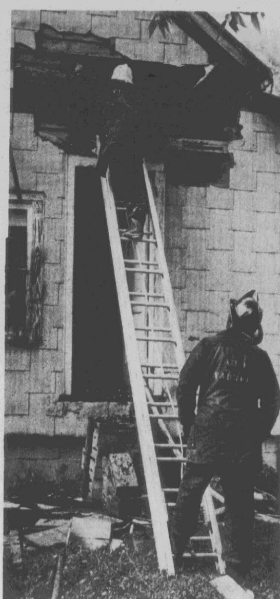
INSPECT FIRE SCENE . . . Firemen check out the attic of a house at 807 Fleming St. which was damaged by fire early yesterday afternoon. Greenville Fire Department officers reported the blaze, which burned the ceiling out of a room at the rear of the dwelling and damaged the attic, apparently started in the attic of the wood-frame dwelling. The blaze was reported at 2:50 p.m.
