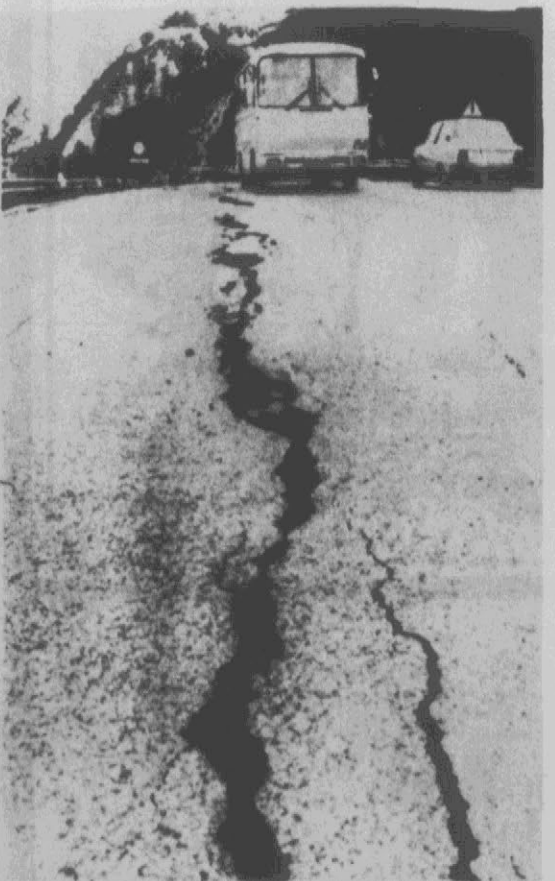
QUAKE-CRACKED ROAD — A crack, several inches wide, and others are clearly visible on the asphalt of a highway at Venzone, in Italy, after new strong tremors hit northern Italy last week. (AP Wirephoto)
