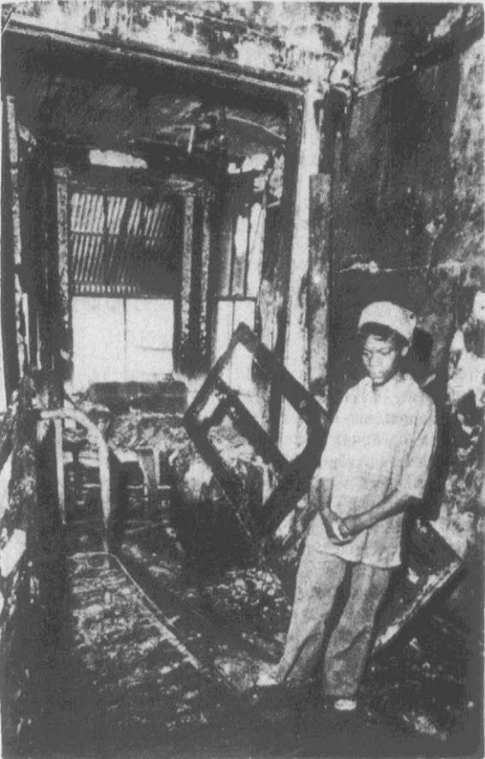
DEATH SCENE—Della Owens, 13, stands in ruins of her second floor apartment on Chicago's Southwest Side where a fire killed seven people including Della's mother and four of Della's brothers and sisters. Two other children died in the blaze which swept through the second and third floors of the building. (AP Wirephoto)
