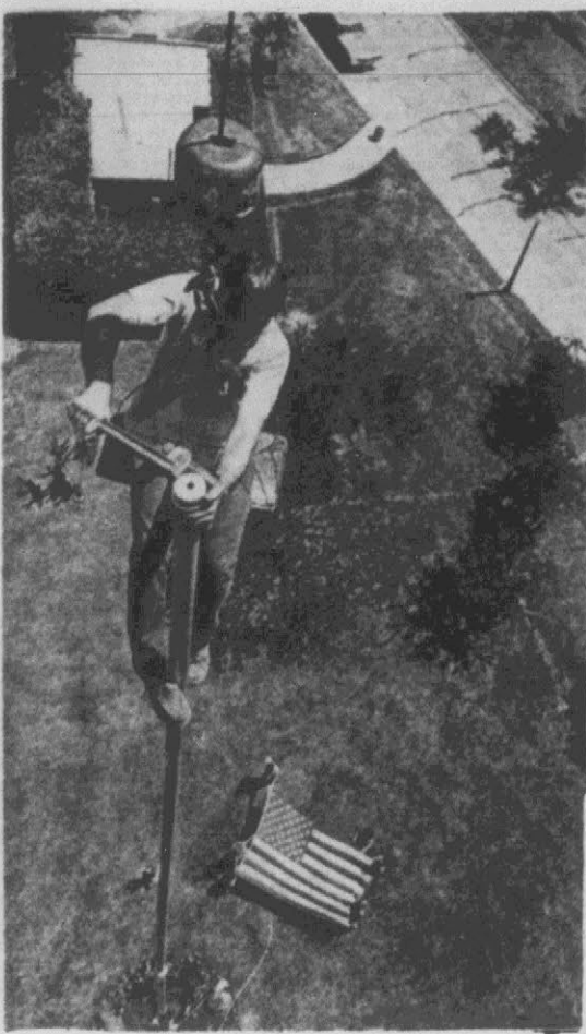
TIP TOP JOB —The 56-year-old flagpole at Greenway Park in Dallas receives some lofty repairs from Jerry Roberts. The neighborhood had the 84-foot pole—one of Dallas' tallest—refurbished for their Independence Day Parade on Saturday. (AP Wirephoto)
