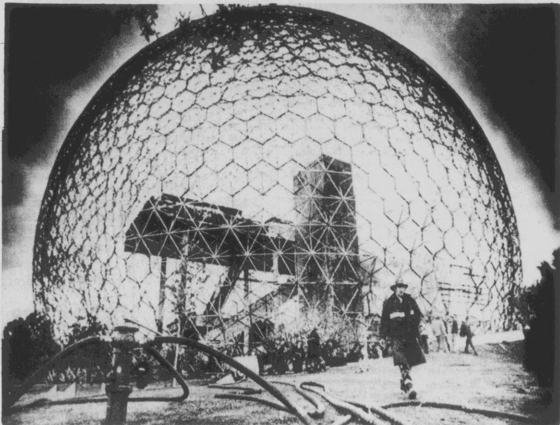
FORMER U.S. EXPO PAVILLION DESTROYED — Firemen mop-up at the former United States pavillion at the Expo '67 site in Montreal after a flash fire destroyed the geodesic dome's acrylic skin, leaving only the aluminum skeleton remaining. One man is missing following the fire. (CP Wirephoto)
