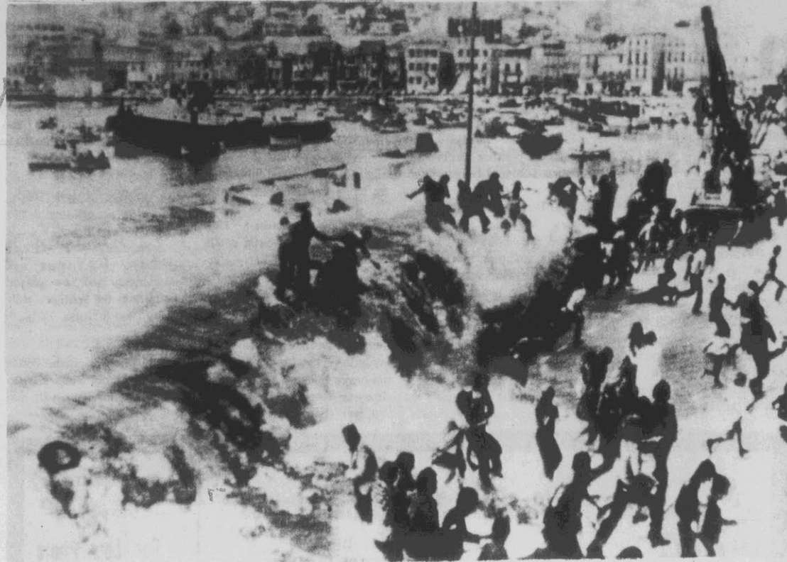
LAUNCHING WAVE —A mini-tidal wave washed some people off a quay as others flee the water at Mediterranean harbor of La Ciotat, near Marseille, Tuesday as the launching of liquid gas tanker
