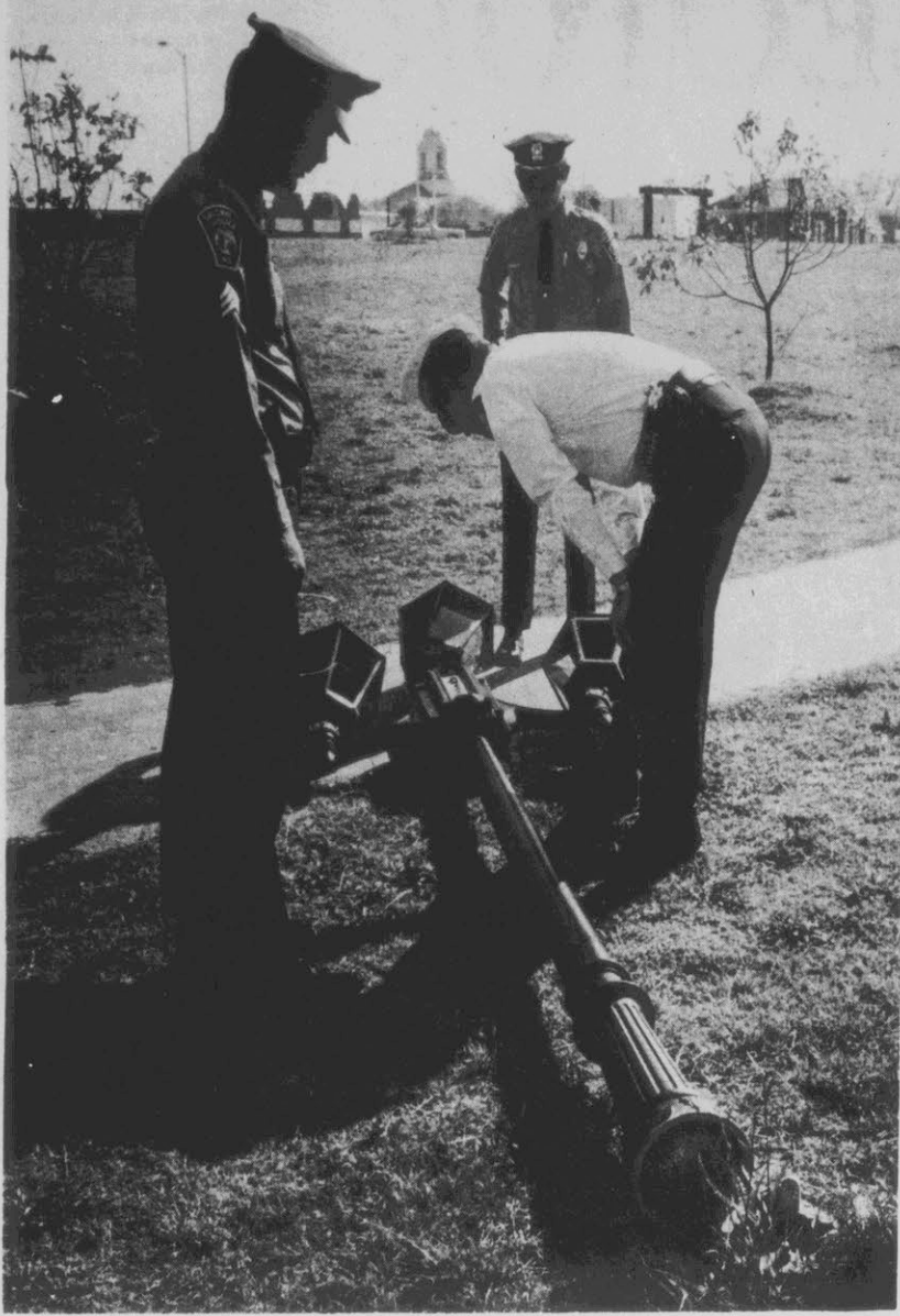
HIT AND RUN VICTIM — Three Greenville Police officers inspect the damage of one of two lamp posts which was knocked over on the Greenville Town Common Sunday afternoon allegedly by a hit and run driver.
