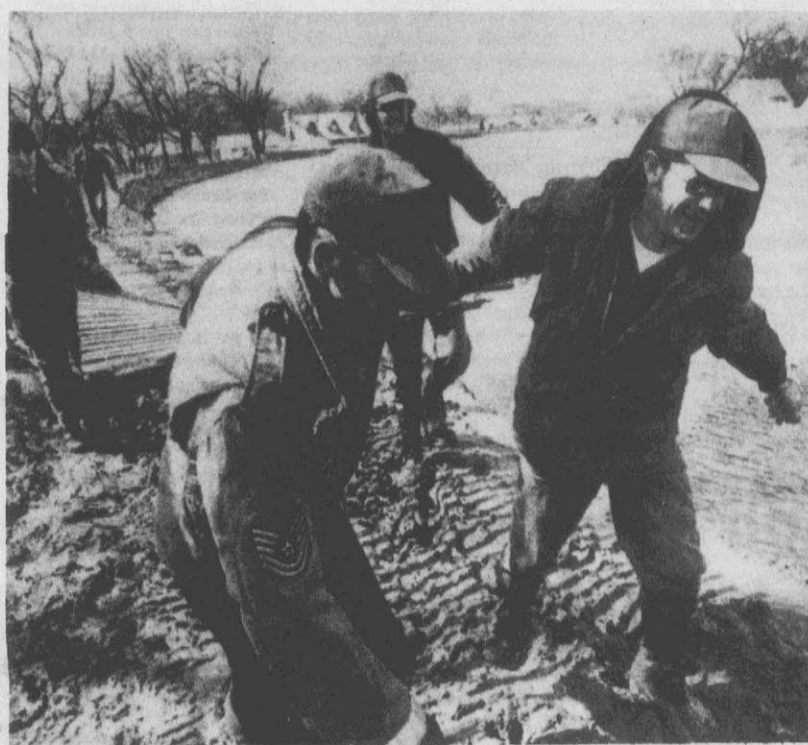
STRAIN —Men from the Minot Air Force Base strain as they pull picket fence across earthen dike to be used to reduce erosion from the high and fast Souris River Sunday. The river crested
