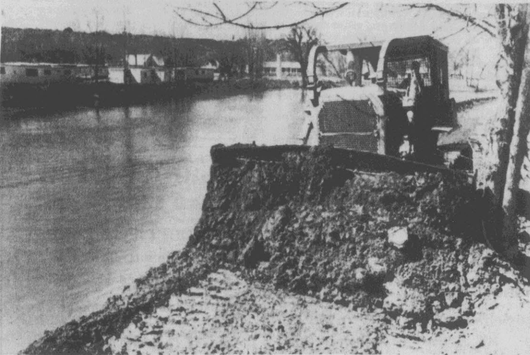
DIKING OPERATIONS — Heavy equipment moves earth along a dike holding back the swollen Sours River at Minot, North Dakota. Dike work is expected to be pressed for 24 hours a day for the next
