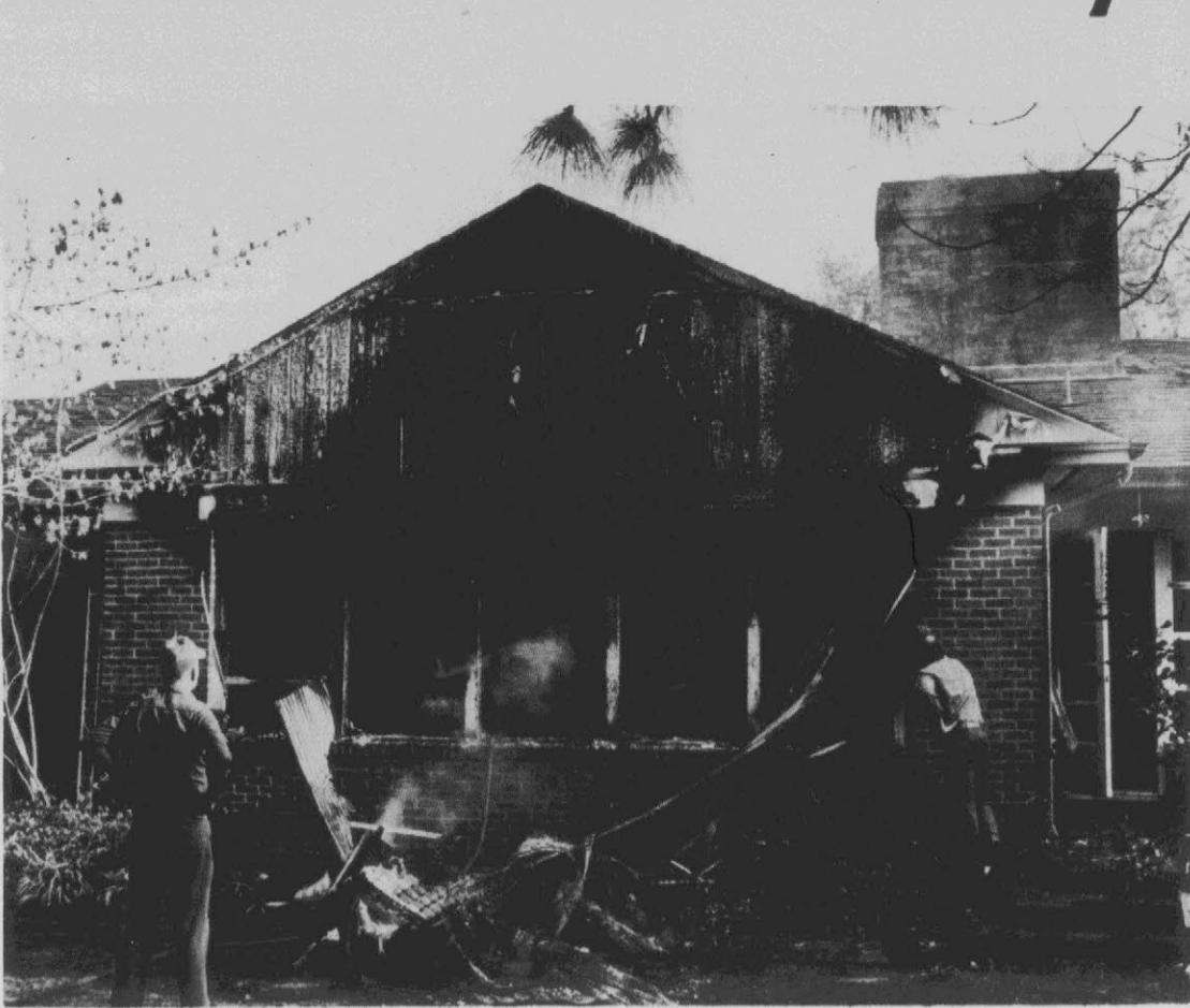
FIRE STRIKES STOKES HOME — Fire severely damaged the Jerome Perkins home in Stokes late Monday afternoon. According to Pitt County Fire Marshall Bobby Joyner, the fire was confined to the den area of the brick home, completely destroying the room. Damages were estimated at $50,000. Smoke and water damage
