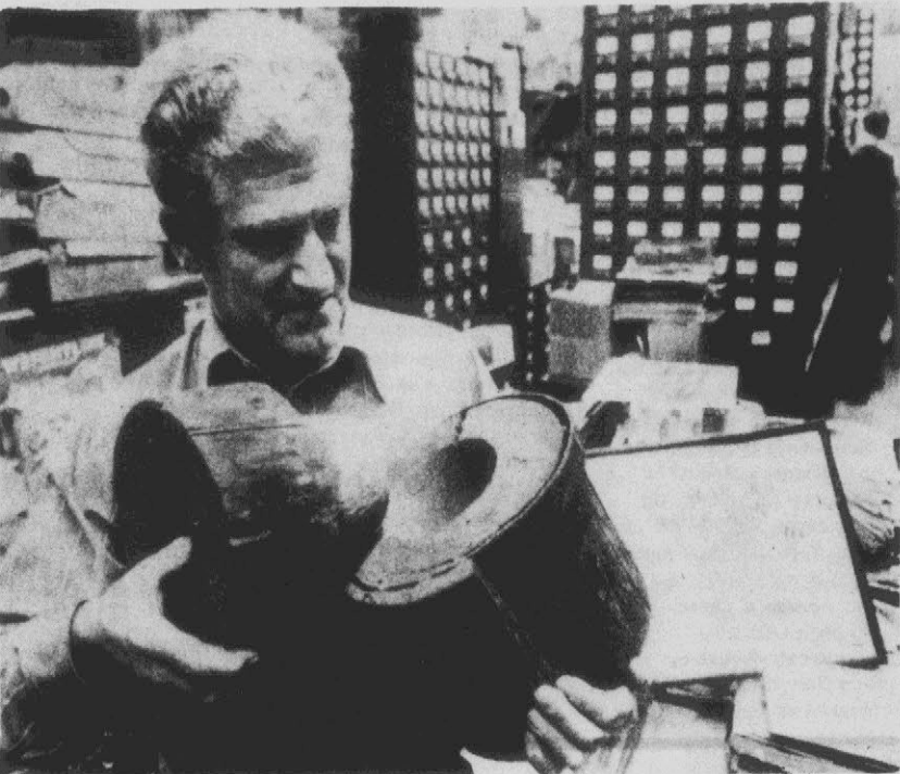
WOODEN WATER MAIN—Jack Gasnick holds in New York a 200-year-old wooden water main, which will go to Washington for use in a bicentennial exhibition. The main, dug up outside historic Fraunces Tavern in New York in 1913,
