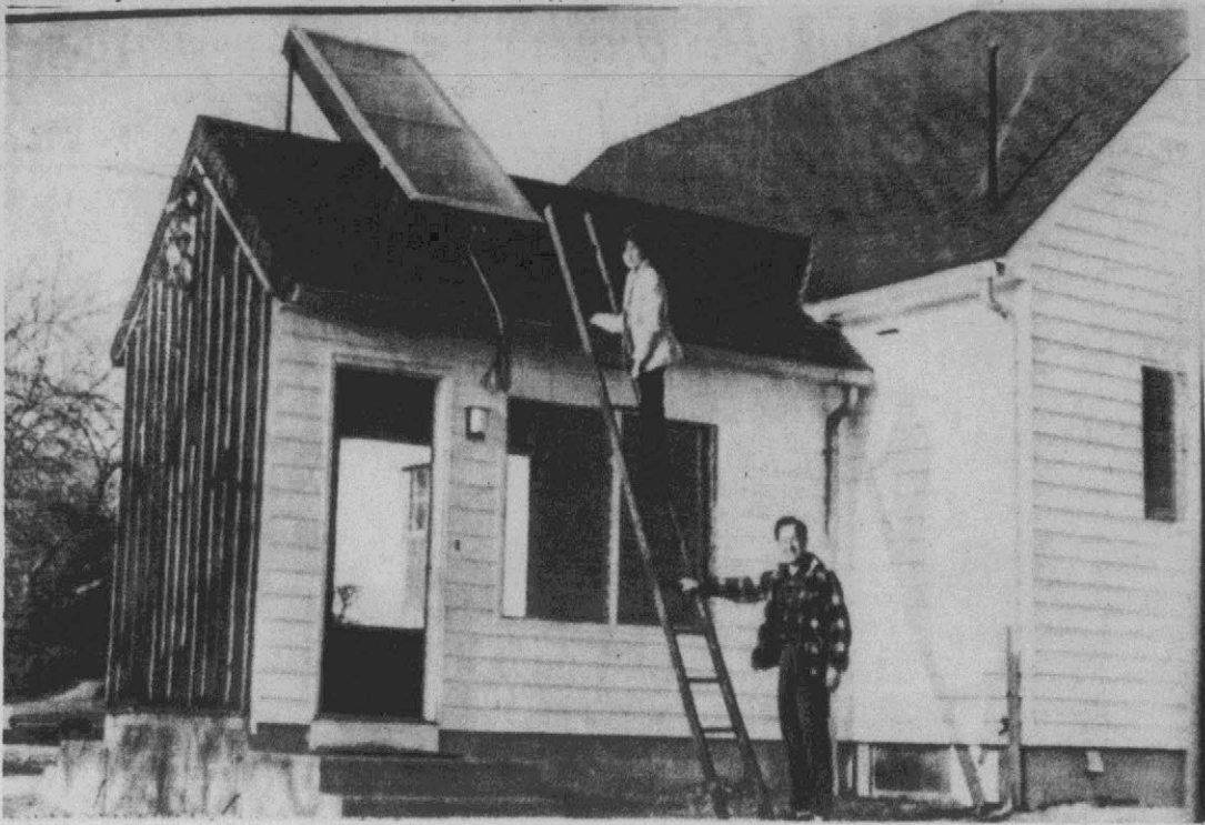
PILOT PROGRAM — Anthony Janovic holds the ladder as his daughter prepares to examine a solar energy unit installed on the roof of their Norwich, Conn. home. The pilot solar energy project is believed to be the first in the nation by a municipally-owned utility.
