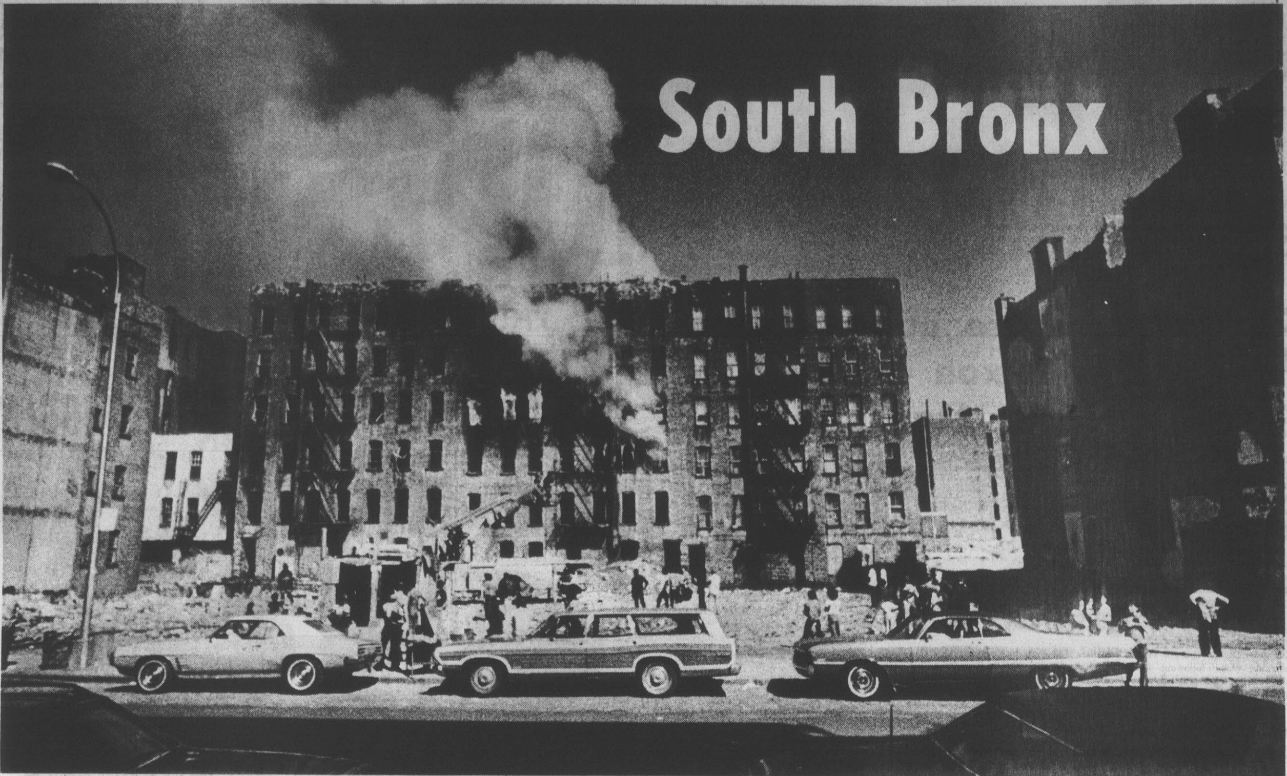
All-too-common occurrence in New York's South Bronx: fire rages through abandoned section of row of houses on partly razed block.
