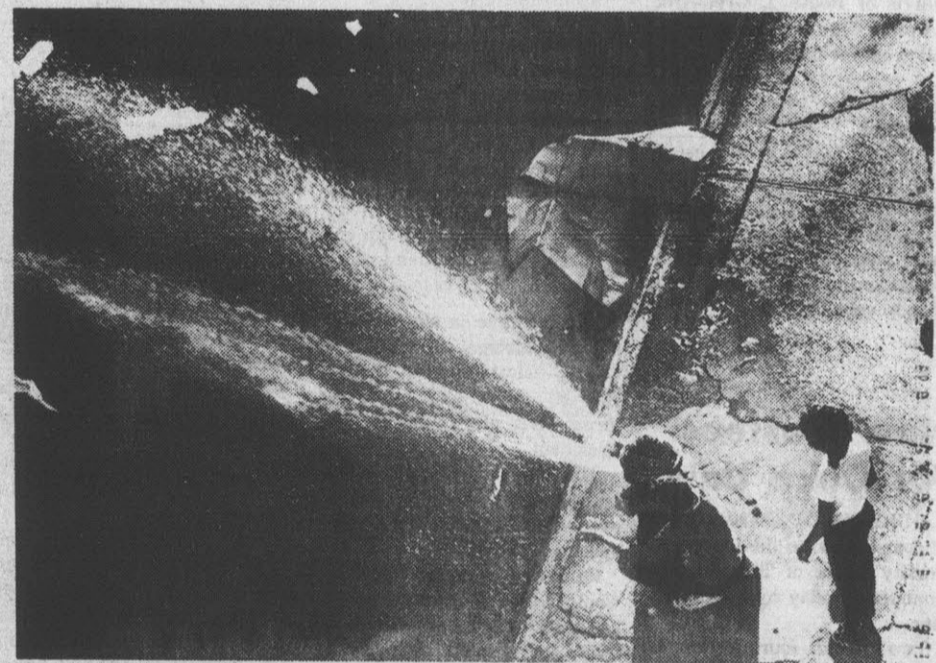
Open fire hydrant provides entertainment for two kids on ghetto street.
