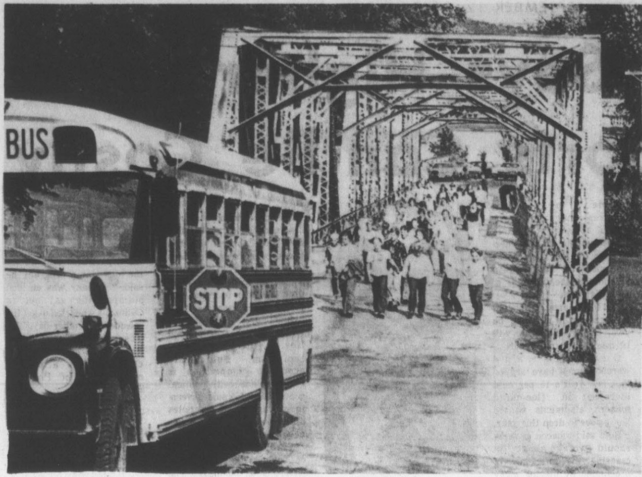
AND LEAVE THE WALKING TO US—School bus waits for La Farge (Wis.) students as they walk across bridge which local school board says is no longer safe for heavy vehicles. The board
