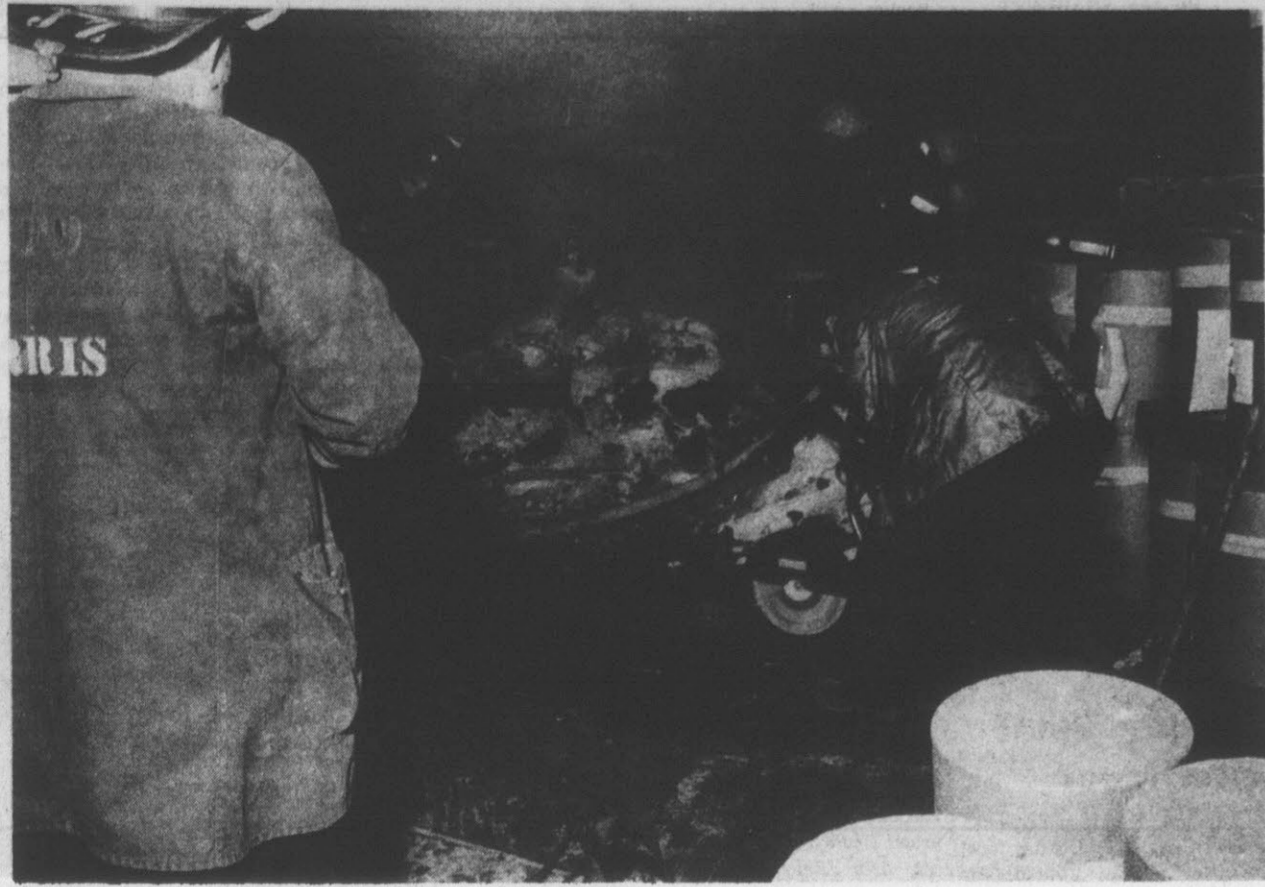
FIRE DAMAGES LOADING AREA . . . Firemen use a portable saw to cut through the flooring at the rear
