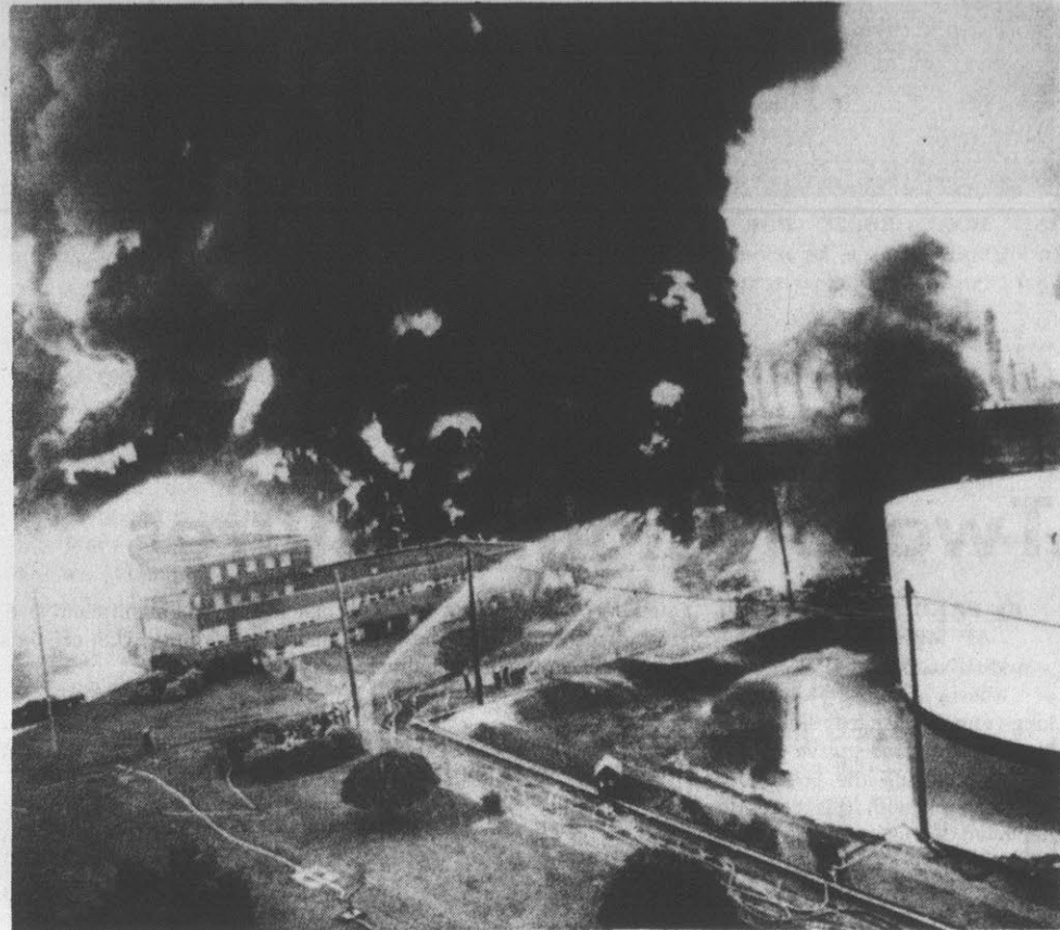
REFINERY FIRE—A multi-alarm fire that started early Sunday morning at the Gulf Oil Refinery in Philadelphia and was declared under control erupts again later in the day. Several firemen were reported missing and three are known dead. (AP Wirephoto)
