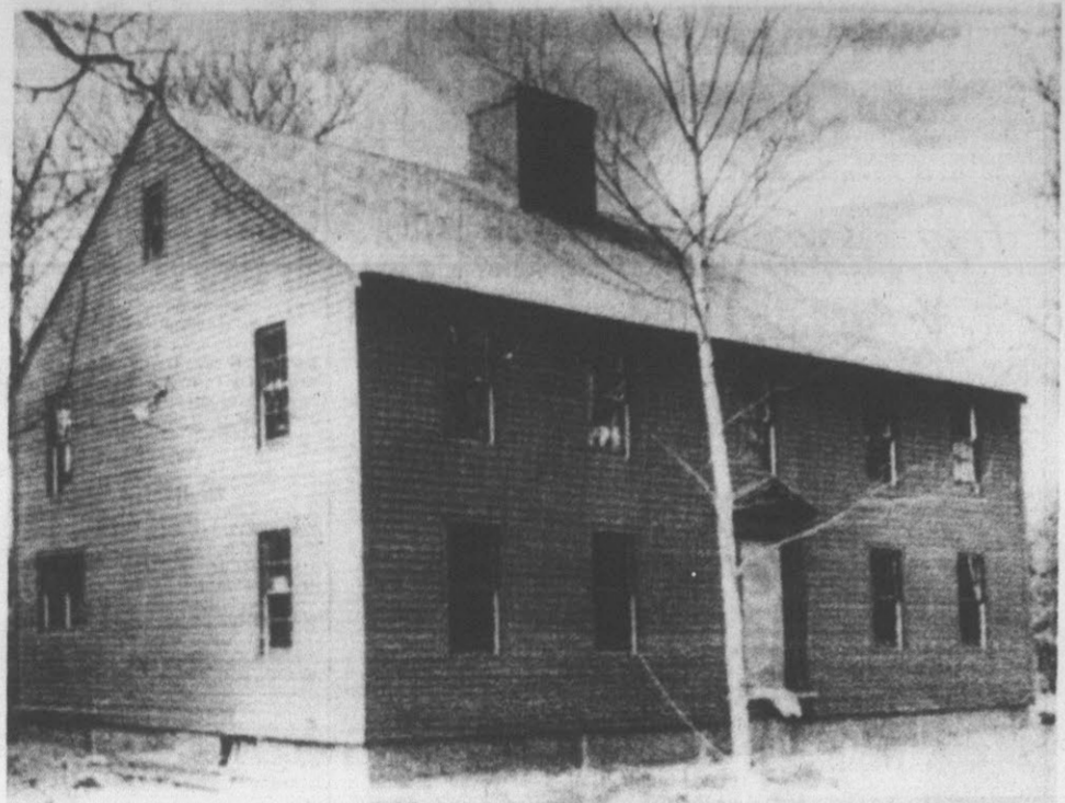
BUILDING THE OLD WAY— Carpenter Stewart Elliott of York, Maine, uses an old broad hatchet to make a dovetail joint in a beam for a timber-framed house. Below: the finished product. (AP Wirephoto)
