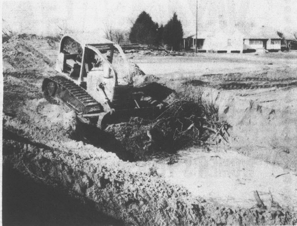
FARM CLEARED. . . A bulldozer is being used to bury debris as the Briley Brothers clean up a farm near Tripps Crossroads they have recently purchased. Old buildings, junked automobiles,
