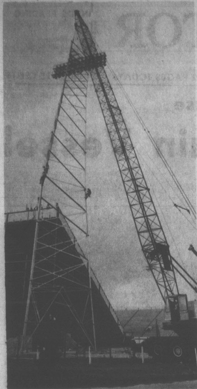
LIGHTS, ACTION FOR THE CAMERA —One of the six new light towers at Ficklen Stadium is swung into place by a huge crane yesterday on the East Carolina University campus. The towers, some 100 feet high, are being completed this week. Four were put into place yesterday and the rest are scheduled for today. The six towers with their banks of lights will make Ficklen one of the best lit stadiums around, allowing the color-casting of games at night. (Reflector Photo)
