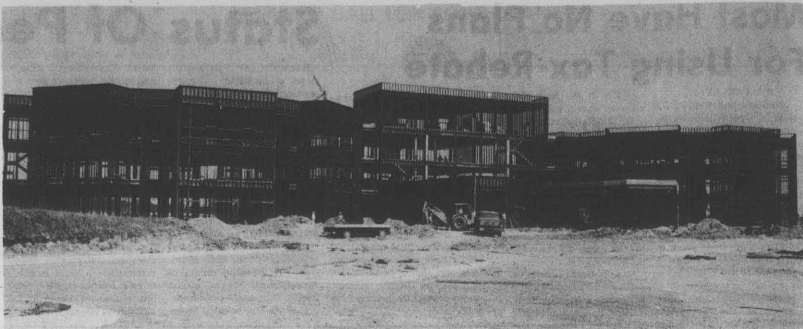
MAKING PROGRESS—Construction on the new Pitt County Memorial, according to hospital administrator Jack Richardson, is about 33 percent complete. The view above of the new facility is a front view with approximately all of the
