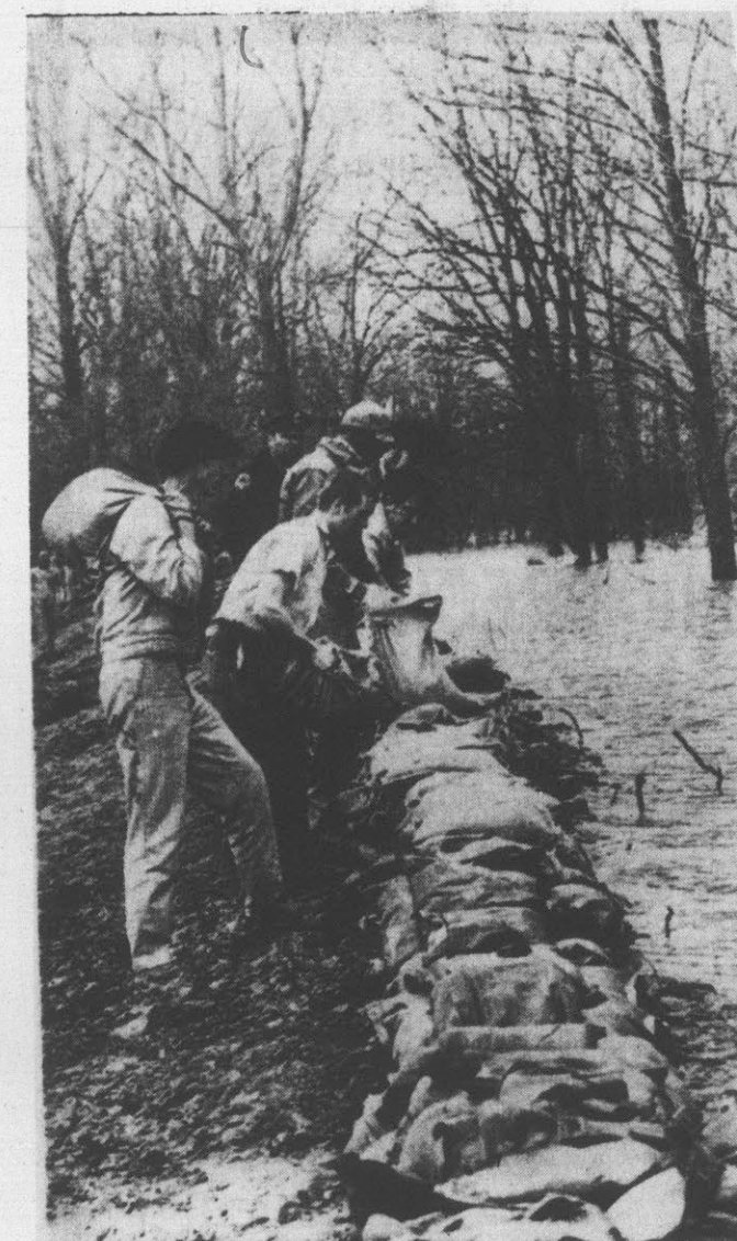
SANDBAGGING—A guard (background) looks on as prisoners from Fort Pillow State Prison are pressed into service sandbagging the Dyer County Little Levee near Dyersburg, Tenn. The secondary levee protects 40,000 acres of West Tennessee farmland situated between the rising Mississippi River and the U.S. Army Corps of Engineers' mainline levee. (AP Wirephoto)
