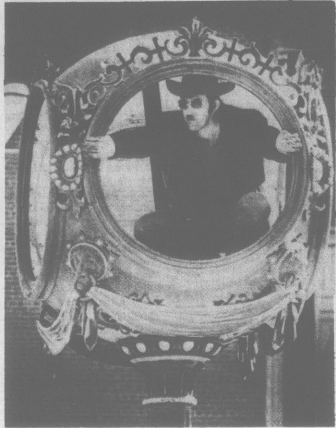
HE'S JUST IN TIME—Doug Parkin works inside historic clock on Salt Lake City's Main Street. It's not known when the clock was erected, but 1868 photographs show the street without the clock, while 1880 photos show it in place. The clock, its pedestal made of bronze and iron, was first run by a waterwheel, then by springs and batteries, then was connected to a master electric system inside a nearby bank. Parkin isn't dismantling the old timepiece for good—it is going into storage until the city completes its Main Street remodeling project. (AP Wirephoto)
