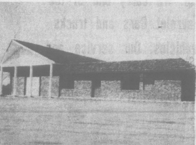
NEW BUILDING . . . The new Living Water FWB Church building will be dedicated Saturday night.
