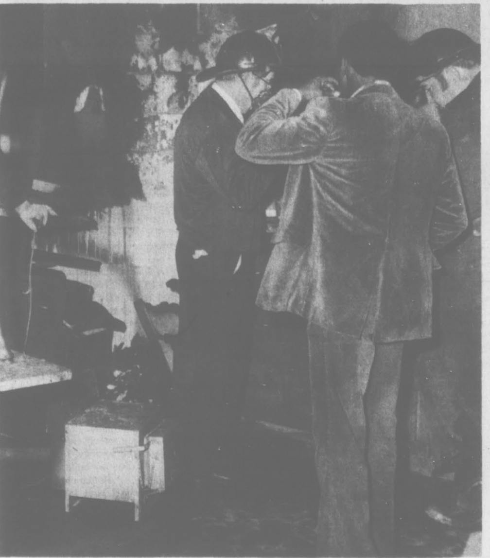
FIRE DAMAGES ART ROOM . . . A fire was contained to the art room on the Rose High School campus last night causing some damage. Investigators above look over the scene. (Reflector Photo by Tommy Forrest)
