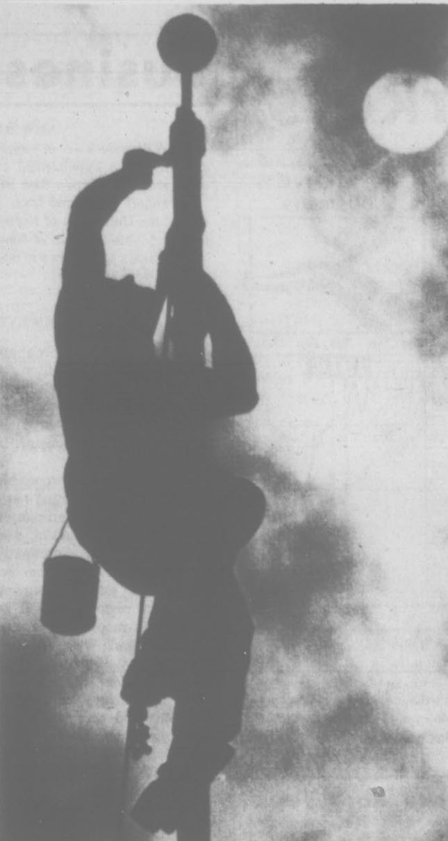
HIGH MAN ON THE POLE —Gerald Ogg is a professional painter, of flagpoles. Shunning ladders and other conventional equipment Ogg has his own method for ascending. A harness with knots that will slide up the pole, but not down, hold him in place while on the job. Ogg has traveled all over the Southeast as a painter of flagpoles and finds the work refreshing and alleges that he always works with a beautiful view in sight. (AP Wirephoto)
