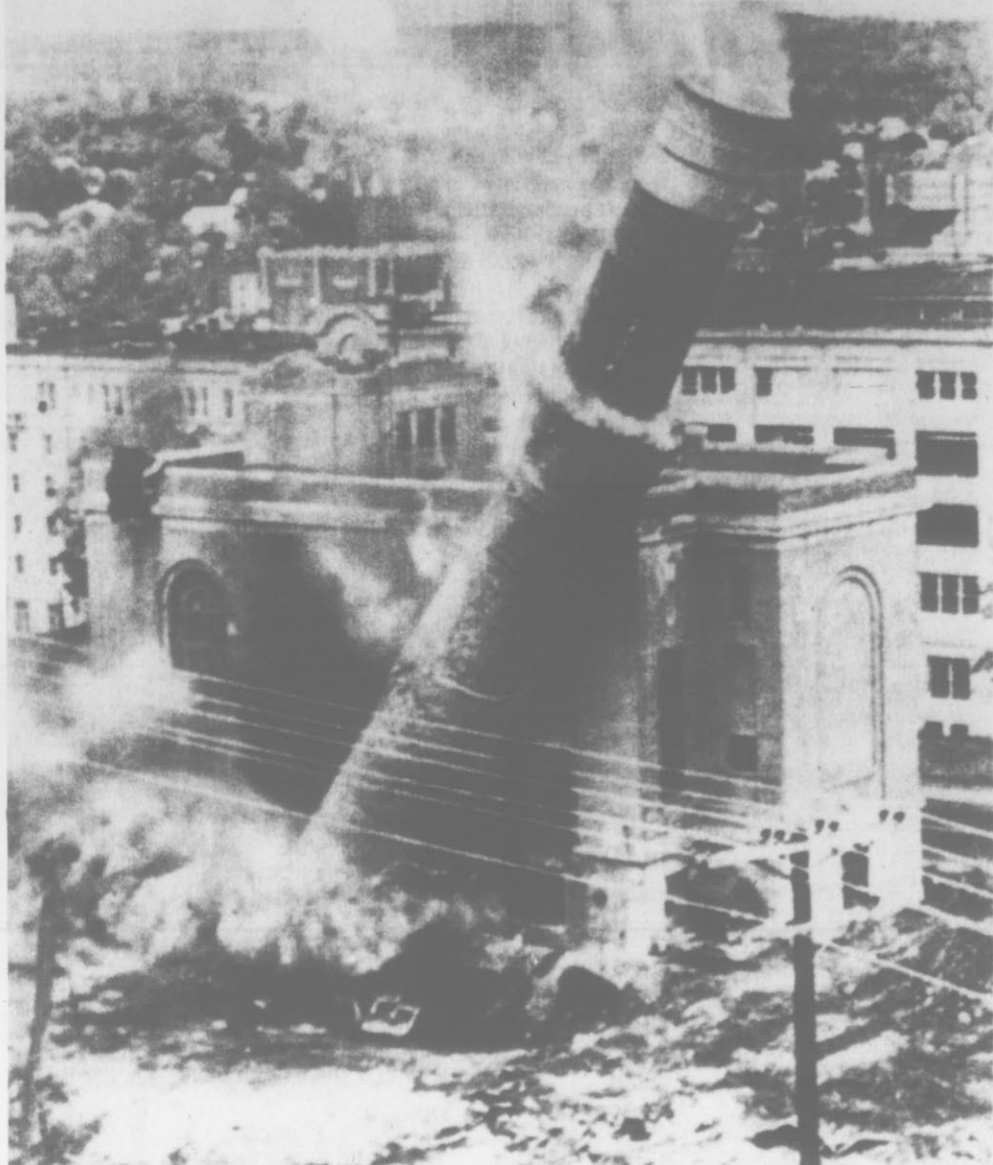
LEANING TOWER OF BRISTOL—A 210-foot smokestack at the New Departure Co. power plant topples Sunday morning in Bristol, Conn., after workers set off explosives to bring it down. The tower was removed as part of a redevelopment project. (AP Wirephoto)
