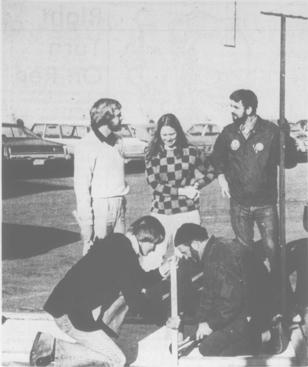
A NEW JAIL...for Greenville was started late Thursday afternoon as volunteer construction people gathered at the corner of Fourth and Evans Street. Shown at work are (kneeling, left to right), John Anders of Havelock and Emmett Peaden, Greenville. At back, Houston Tucker, (left) Greenville and Adrian O'Neal, Elizabeth
