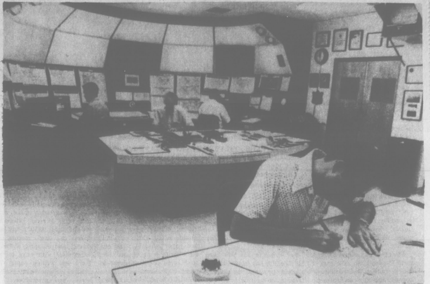
HURRICANE CENTER WAR ROOM—Members of the National Hurricane Center staff stationed in Miami, Fla., follow their familiar routine as they
