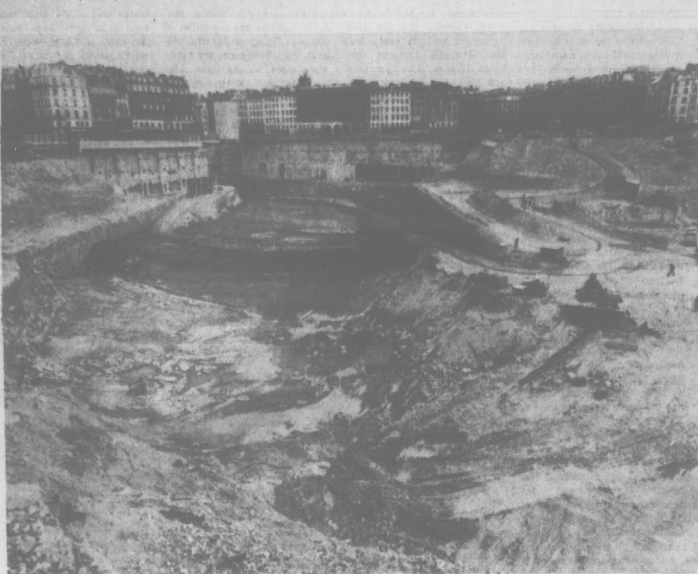
D'ESTAING STEPPED IN—This is the hole dug for a high-rise trade center project which was killed by
