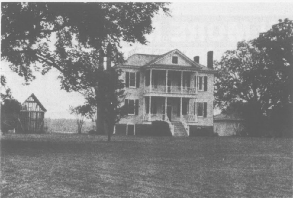
BERTIE'S HOPE PLANTATION... is one of eastern North Carolina's finest early 19th century plantation houses, noted for its Chinese Chippendale balustrades. The framework of a building at left is a smoke-house being restored. (Reflector Photo by Jerry Raynor)
