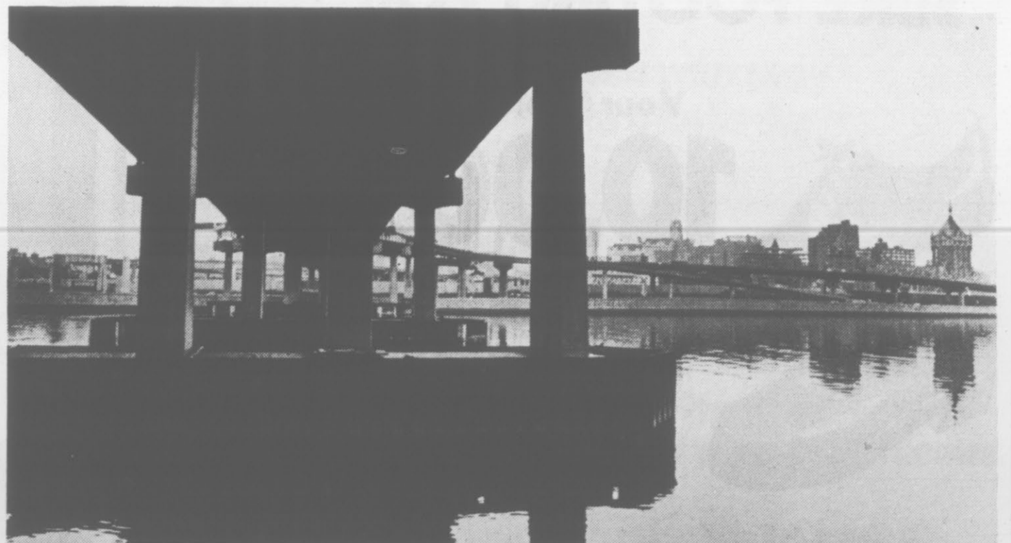
New bridge sweeps combined routes, including Broadway/Old Post Road, into Albany.
