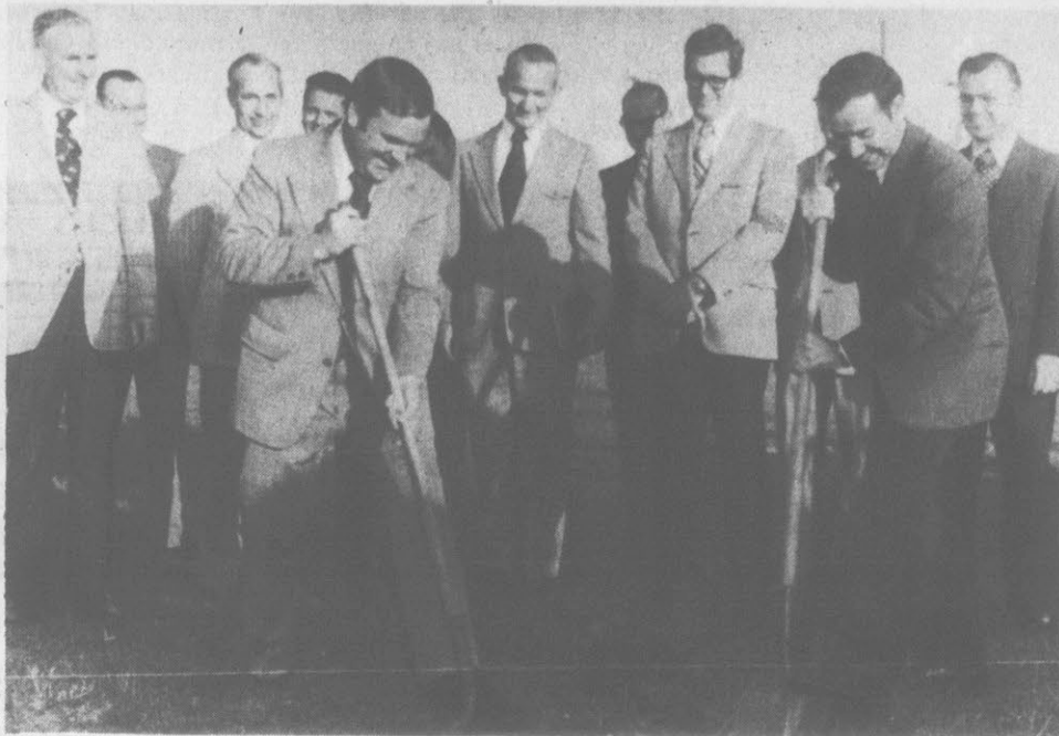
This was the scene at the building site of Trinity's new 1200 seat sanctuary and additional Educational facility. Turning a spade of soil is Pastor Al Davis and James Cobb, a Building Committee member. Looking on are the Deacons, Trustees and members of the Building Committee. Construction is now in progress.
