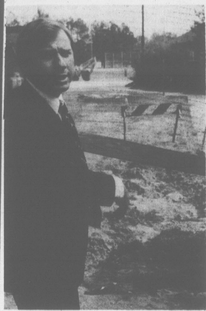
PRINCIPAL'S PROBLEM. Grifton Elementary School principal N.I. Baldree points out the caved in section of his school ground caused by a collapsed sewer line running through the grounds. (Reflector photo by Carl Tyer)
