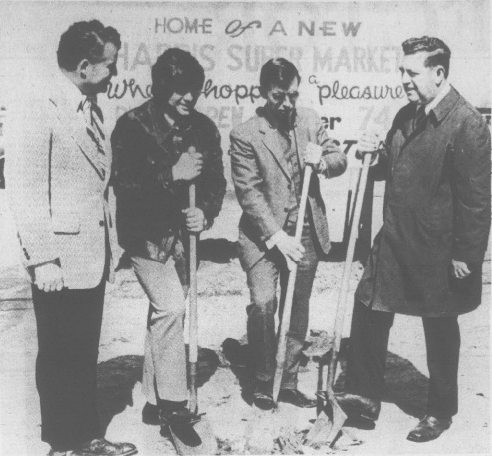
WORK UNDER WAY—Work is progressing on the new Harris Supermarket in Ayden. Participating in the groundbreaking for the new facility recently were (L-R) Durwood Harris, owner; Durwood Harris Jr.; Jack Tyler, manager of Big Value Drugs which will occupy part of the building; and Ralph Ford, Ayden town administrator.
