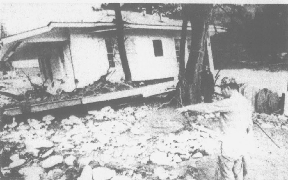
RIVER MOVES HOUSE—Don Wezdenko points to the spot where his house used to be before the worst Sacramento River flood in 50 years swept through the hamlet of Castella, Calif. House came to rest 30 feet away from its original location, lodged in a cluster of trees that kept it from being swept down the river. (AP Wirephoto)
