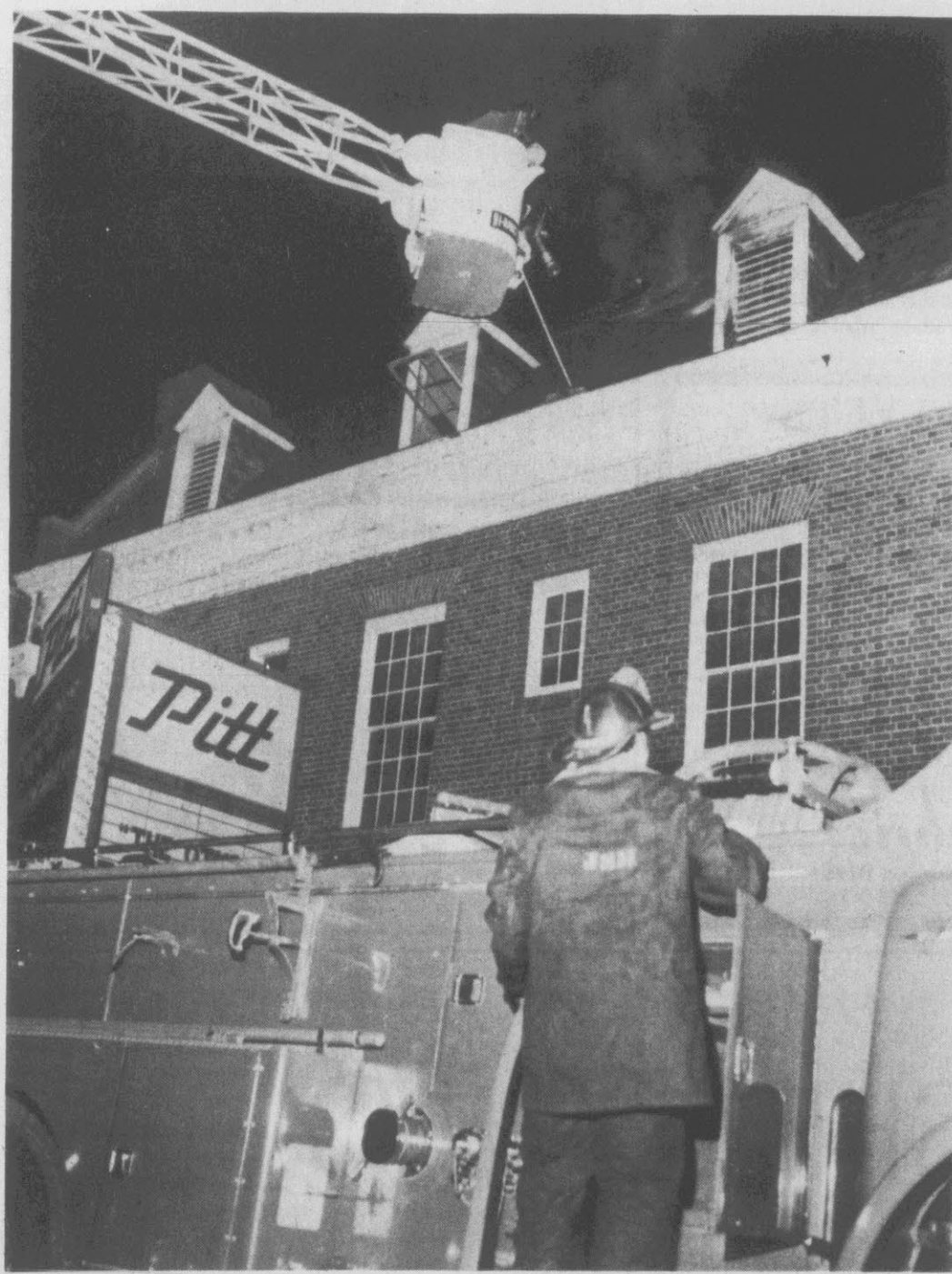
LONG ARM AIDS FIREMEN... Greenville Fire Department's modern snorkle fire engine aided last night in fighting a fire that heavily damaged the Pitt Theatre on Evans Street. Cause of the blaze is still under investigation. (Reflector Photo by Tommy Forrest)
